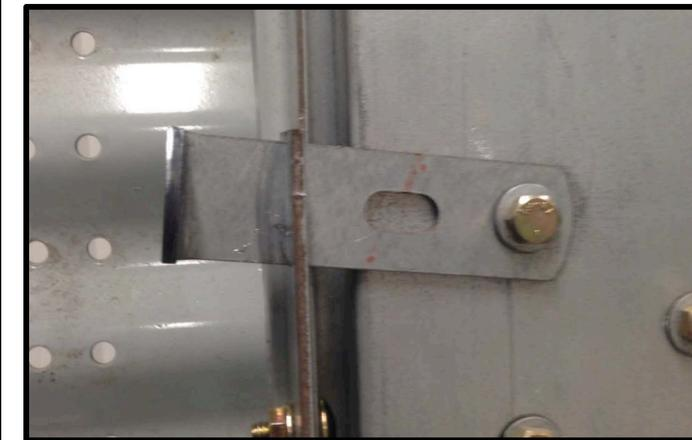
Illustrated here is the current outer door latch design in production from GSI.
